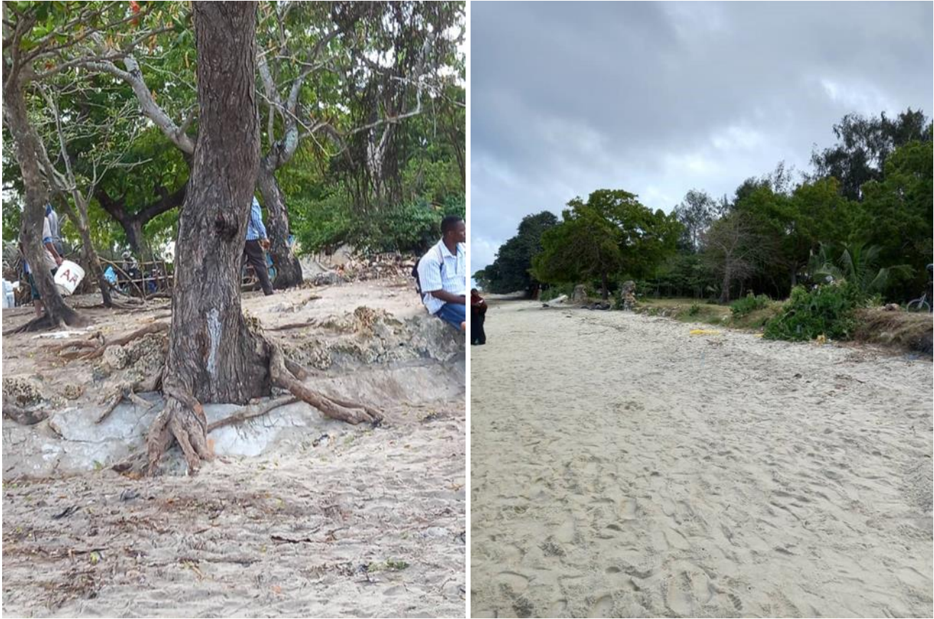
Figure 4. Beach erosion at Kizingo and the remnants of a seawall that provided some level of protection
